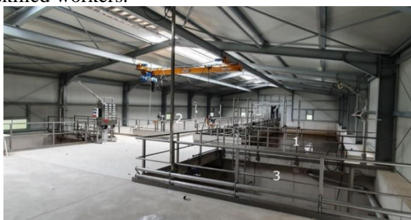
Fig.1. Heringhausen wastewater treatment plant - 1 = SB reactor no. 1, 2 = SB reactor no. 2, 3 = surplus sludge storage (Photo source: J. Wiese)
